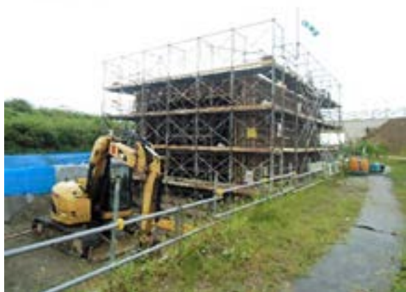
Figure 6. Box culvert building site in Nagaoka
