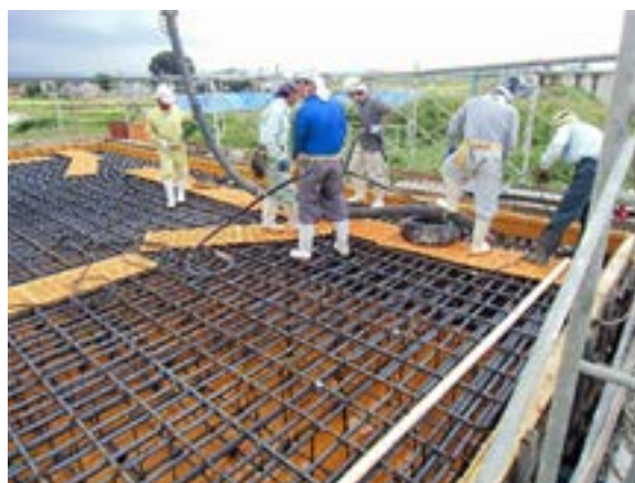
Figure 7. Placing and compaction of concrete
